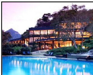
Kandalama Hotel, the First LEED Green Building Outside the USA and the First LEED Green Hotel in the World; 2000
