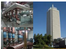
Dubai World Trade Center Sheikh Rashid Tower
